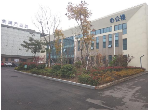
厂区内绿化现状 (2024.12)
