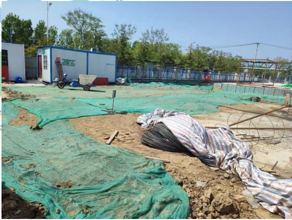
裸露地表密目网苫盖
