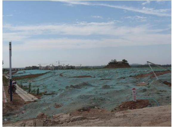
厂区密目网苫盖
